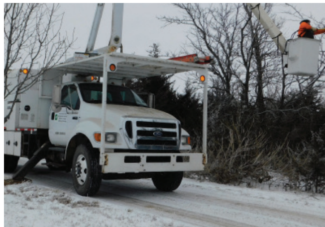
Having trees near power lines trimmed professionally prevents limbs from falling on power lines. Sedgwick County Electric Cooperative contracts with Ashley/Ingram & Sons to clear cooperatives right-of-way clearances.
